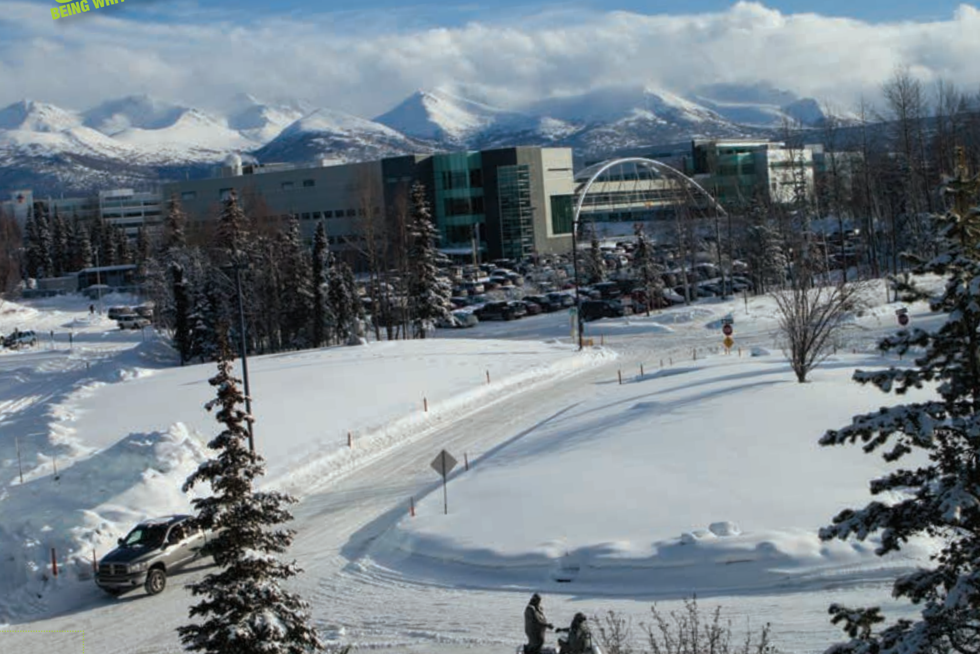
Set against a backdrop of the Chugach Mountains, the Parrish Bridge spans Providence Drive to connect the Engineering & Industry Building (EIB) and the Health Sciences Building. Alumnus Mike Fierro, B.S. '89, M.S. '01, served as lead structural engineer for the EIB and also designed the Parrish Bridge, named in honor of longtime university supporters Ann, B.B.A. '78, and Al, Honorary LL.D. '12, Parrish.
