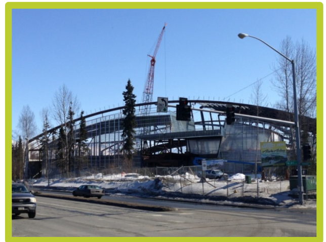
Alaska Airlines Center, Construction Underway
