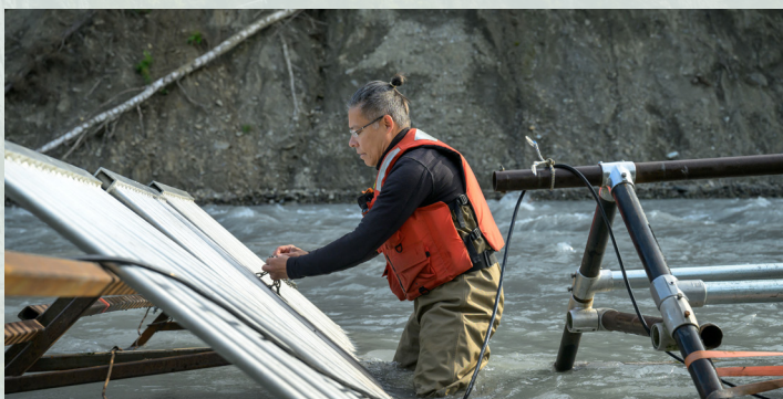
AERC Research Technician John Naumann adjusts the fish weir in Eagle River. Russo and his welding students built the weir specifically for AERC.
