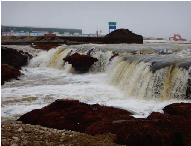
Water overtopping the Dalton Highway near Deadhorse during Spring 2015
