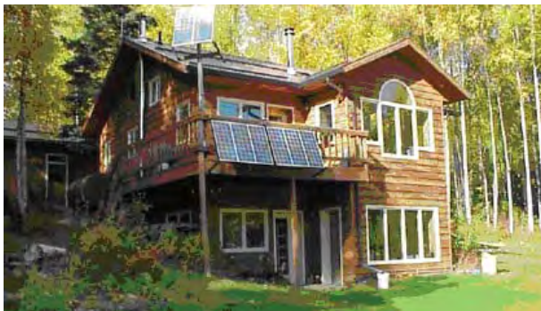
This home near Fairbanks uses a combination of photovoltaic cells for power, an active solar water heater, and passive solar design.
